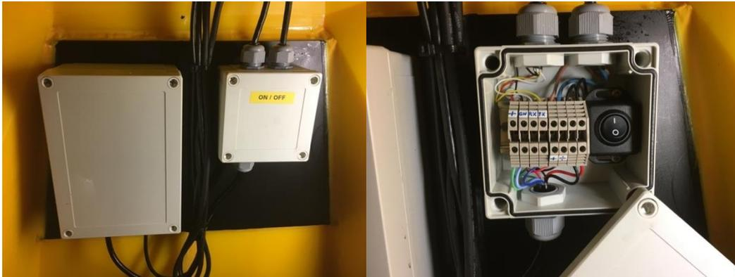
Figur 6-Power switch box inside the buoy.
